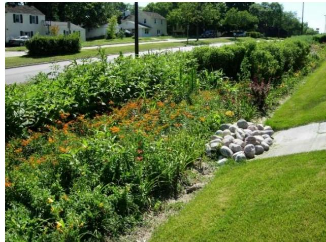
sand/ gravel or other well-draining subsoil, below a deep, well-draining growing medium. Above this there is a ponding area of variable depth and a high-level discharge pipe or spillway. The figure opposite is an example of a bioretention zone. Trees, shrubs or other vegetation can be planted in the bioretention area as required. Below is a typical cross-section of a roadside bioswale.
