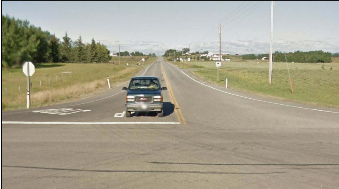
Figure 4: Minor Road Approach with Informal Right Turn Lane (Cochrane Lake Road at Highway 22)
